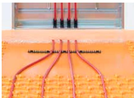
The levelling panel Schlüter-BEKOTEC-ENFGTS is installed in front of heating circuit distributors to simplify the heating pipe installation in the distributor cabinet. The polystyrene panel is adhered to the studded panel with the supplied double sided adhesive tape (6 m). To keep the heating pipe securely within the system, the same impact sound insulation is installed under the levelling panel as with EN 18 FTS.
